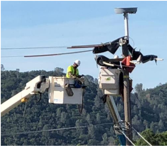
PG&E work crew dismantles a dangerous nest on a power pole near Austin Park in the City of Clearlake and installs an alternate safe location for the Osprey. Photo by neighbor Michael Johnson.
